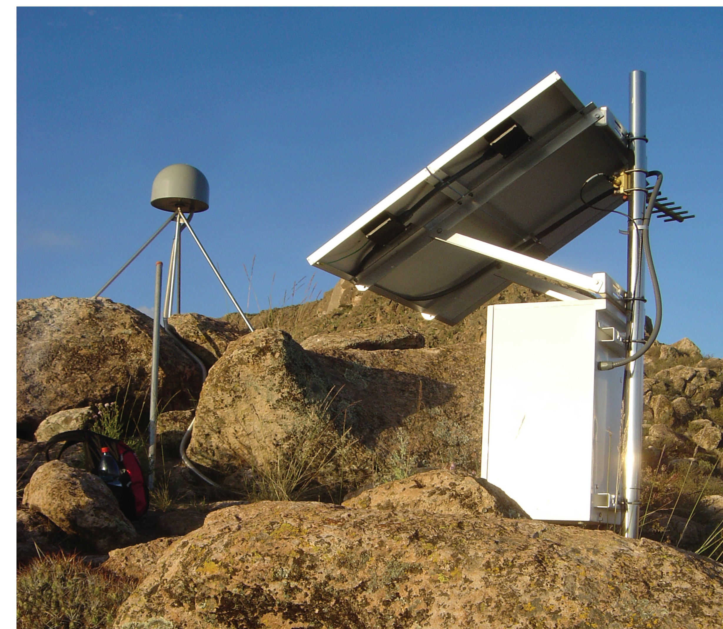
Figure 6. CAGA station PTRE.
