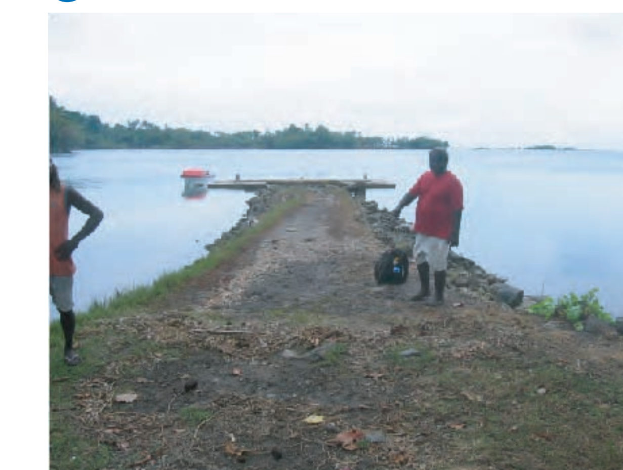
Head man points to new high tide strandline on Simbo, where dock is completely inundated during high tide. Subsidence 0.7 m.
