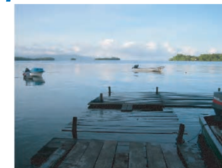
Dock submerged at high tide near Munda. Subsidence 0.6 m.
