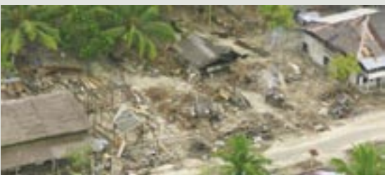
Above: Detail of tsunami damage in a town along the southwest coast of Simeulue.
