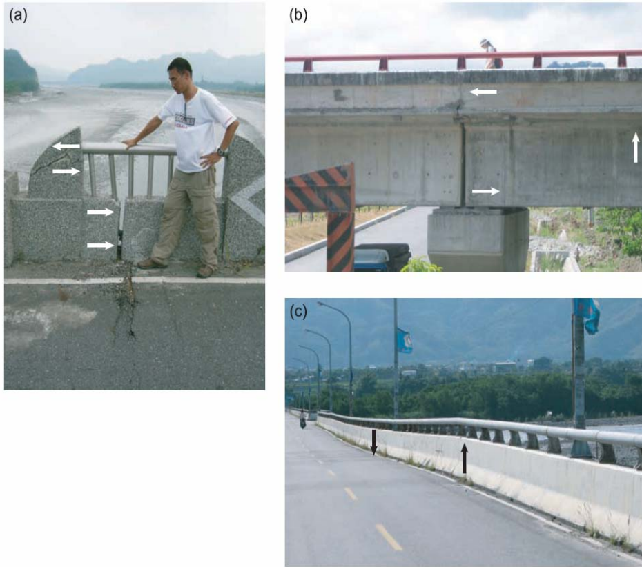
Figure 6. Field photographs of several deformed bridges across the Peinan River. (a) About 200 m from its eastern end, the Luanshan Bridge has been fractured, with its eastern part displaced relatively westward. View is toward the south. (b) Near the eastern end of the Lichi Bridge, an eastern section of the bridge appears to have moved upward and caused deformation of its contact with its neighboring section to the west. The lower part of the contact appears to have opened and the upper part of the contact appears to have narrowed. View is toward the north. (c) About 100 m from its eastern end, the Paohua Bridge has been deformed by the Longitudinal Valley fault. The eastern part of the bridge has moved upward with respect to its western part. View is toward the west.
